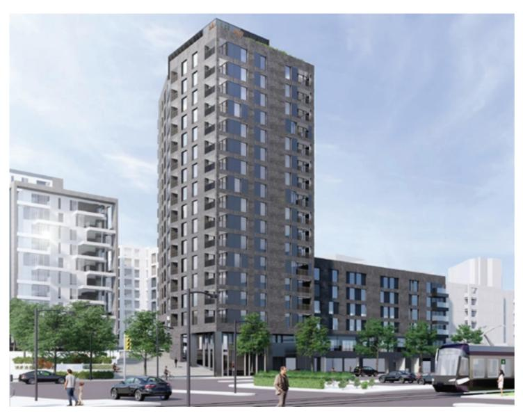
Study 1: 3D visualisation showing an elevational treatment consisting of dark brick walls and columns in the corners. The communal multi function room at the top is set back. This option was discarded in favour of the approach shown in study 2.
