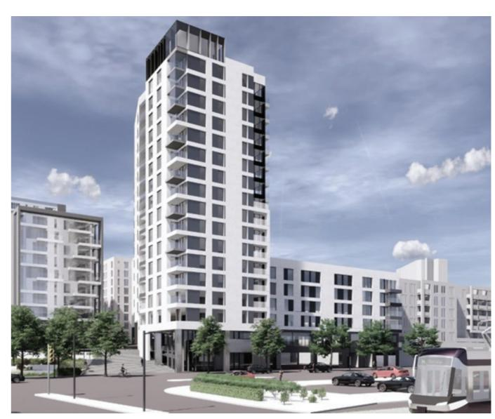
Study 2: 3D visualisation showing a light coloured brick, with the communal room crowning the building at its corner. A double order treatment in the balcony cladding is used as a device to make the corners lighter, thus increasing the perception of slenderness.
