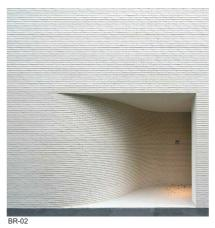
BR-02 Selected Brick or brick panel system with white tone colour, light colour mortar joint to match, raked
